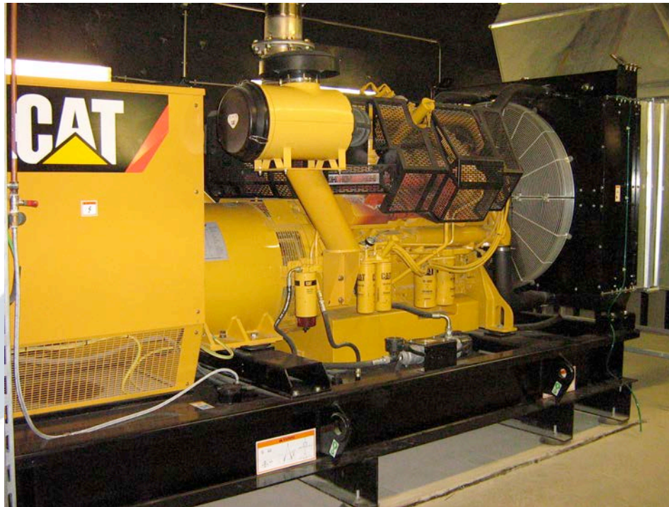
2 Diesel generators at ALBA (720kW each)
