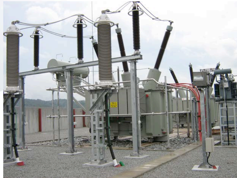
220 KV/25 KV TRANSFORMER
