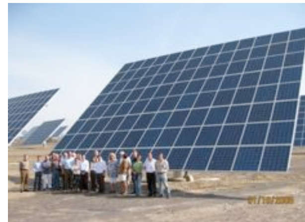
Nearby the Moura Solar Photovoltaic plant. generating over 60MW with 350.000sqm solar cells over 1000 solar trackers,
